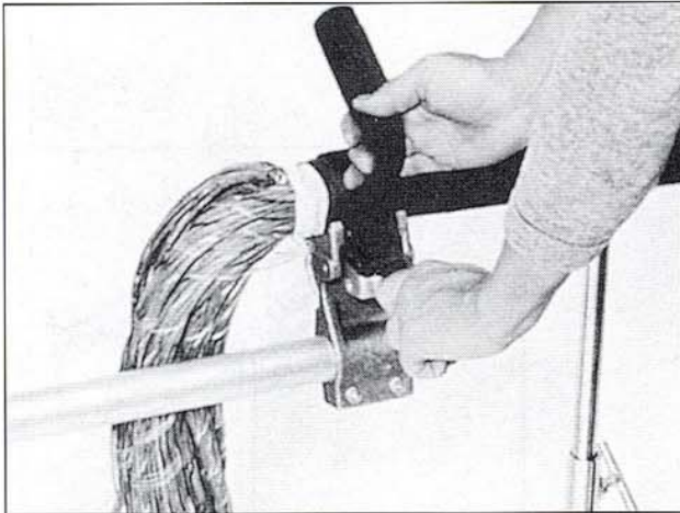
Pull the strap tight and push the latch down to secure the stay tube to the cable.
